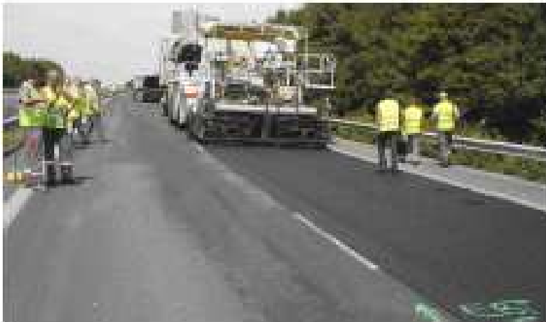
Figure 2: Paving a high-modulus LMA 2 mixture (with 50% RAP aggregate and with a new 10/20 mm grade source) at 10°C on the French A28 Highway and Highway near Paris.
