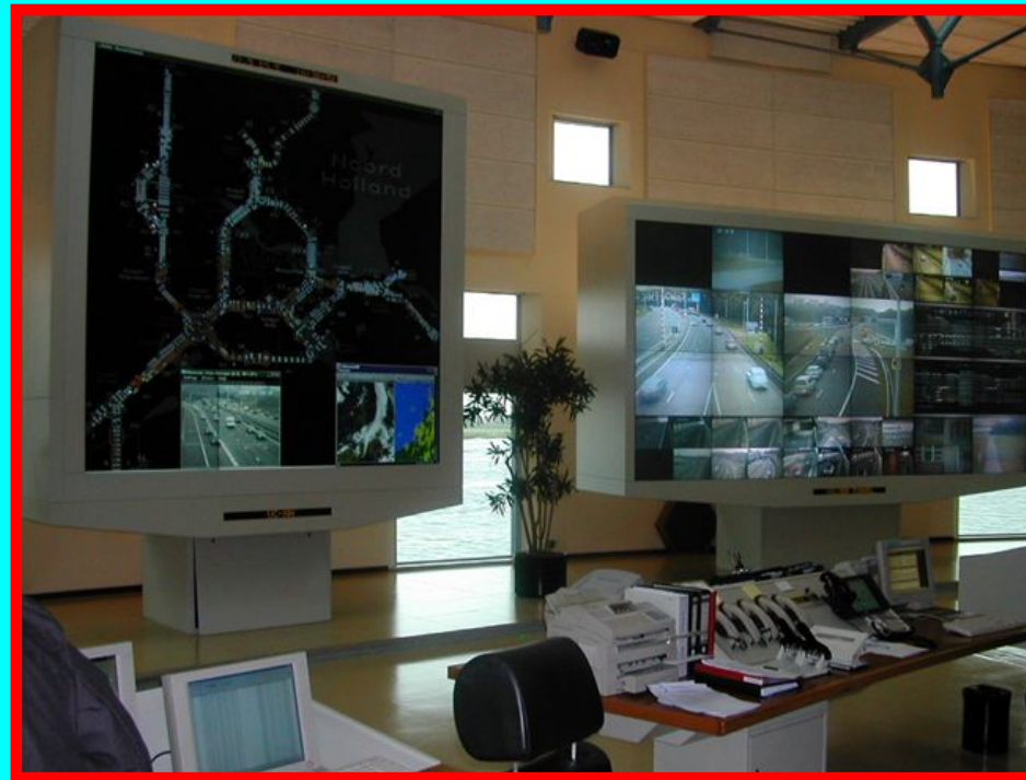
Traffic Control Centre
